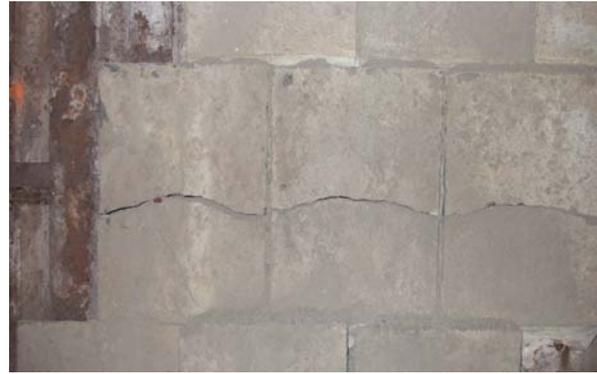
**Figs. 2 and 3** Consequences of the volume expansion of SiC materials in the incineration boiler
