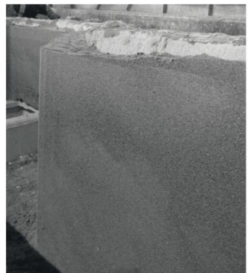
**Fig. 8** Installation of the cold setting mix at GSW Santander
