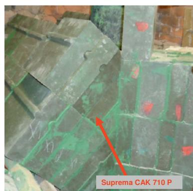
**Fig. 5** Arch area of the post-combustion chamber lined with tongue and groove brickwork during start of installation
