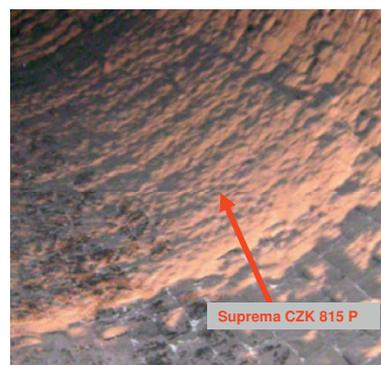
**Fig. 3** Half-shell trial in a rotary kiln
