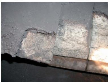
**Fig. 3** Damages of supporting bricks inside a HTR, positioned on alloyed steel-consoles
