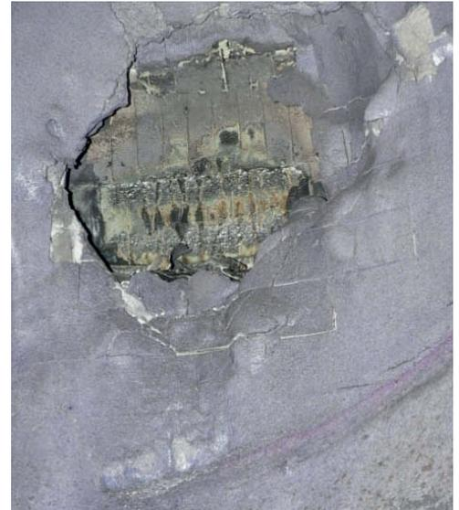
**Fig. 1** Local damage of the hot face brickwork in a high temperature reactor (HTR)
