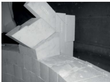
**Fig. 2** Repair by bricklaying with high alumina dense bricks for the hot face and bubbled alumina LW-bricks for the backup insulation
