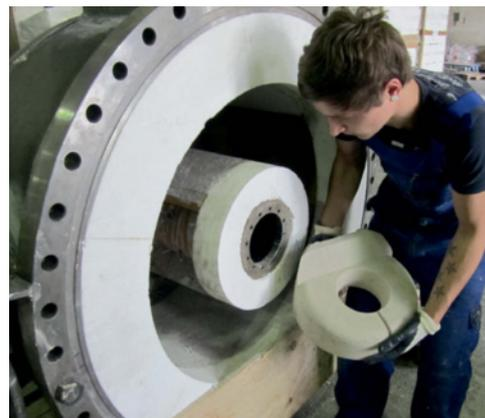
**Fig. 7** Example for the installation of preformed shapes
