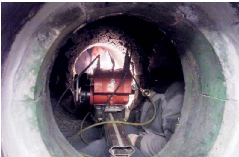
**Fig. 4** Special cutting equipment for careful demolition (especially for dense bricks)
