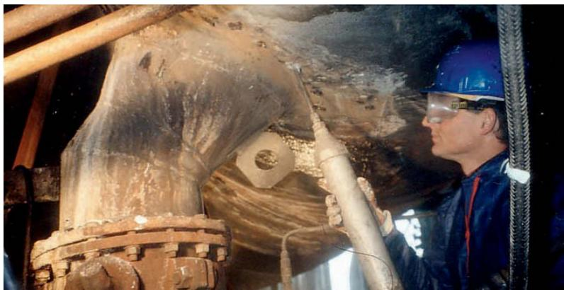
**Fig. 10** Hot spot repair of a BF of a hot blast duct by injection of fibre-mastic with a Quickplaster
