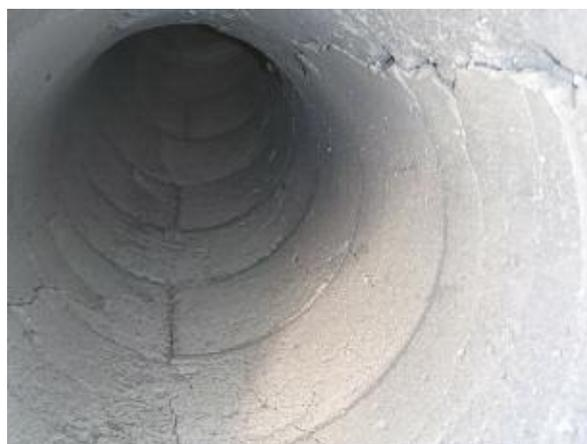
**Fig. 4** Transfer line showing condition of hot face refractory surface
