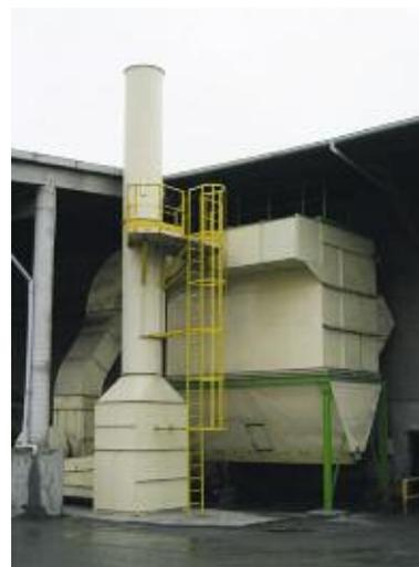
Fig. 7 De-duster serving the mill plant
