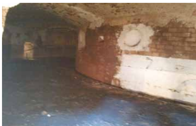
Fig. 4 Condition of relining with developed bricks two years after capital repair
