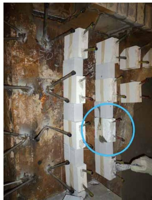
**Fig. 5** Protection shells for steel anchors mounted in an industrial cement kiln [10]
