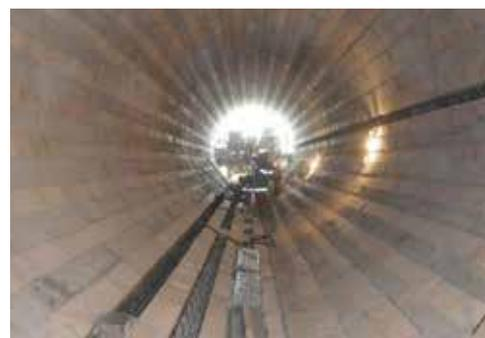
**Fig. 15 Physical assemblage of rotary kiln lining for iron ore sintering**
