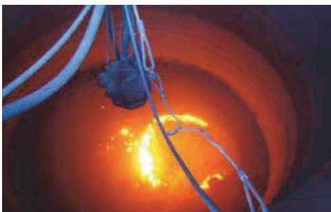
Fig. 2 Robotic shotcrete blast furnace repair at high temperature
