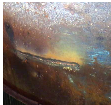
Fig. 2 Example of a horizontal crack at the bottom level
