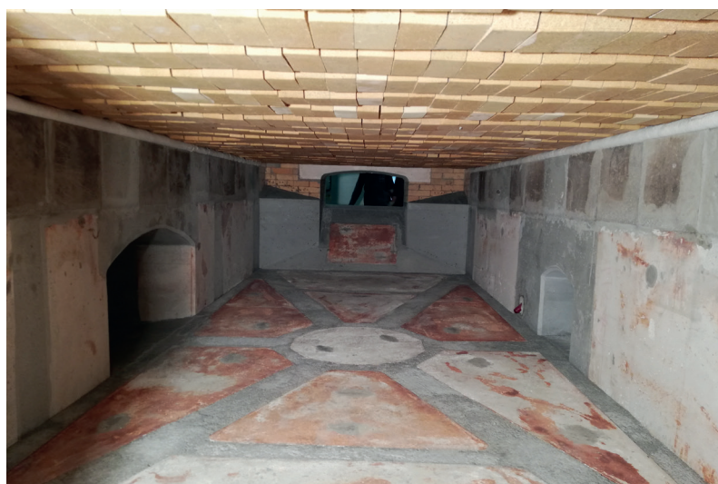
Fig. 3 Lining from the large-format blocks after installation
